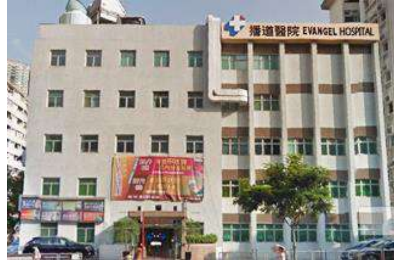
Before installation of elevator
