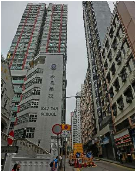
Lechler Court above Kau Yan School
