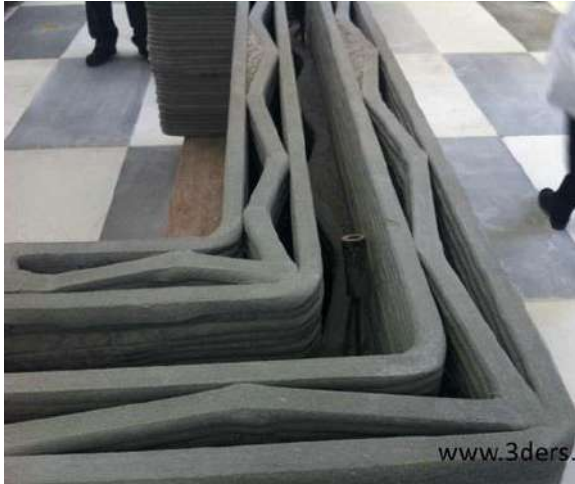
3D printed wall
