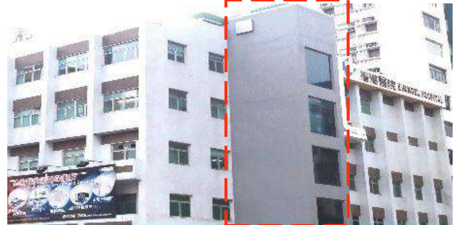
After installation of elevator
