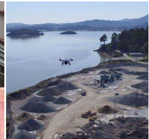
Drone site inspection
