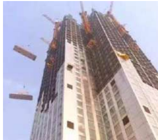
“Skyscraper” at Changsha, China – 57-storey building built in 19 days using prefabrication
