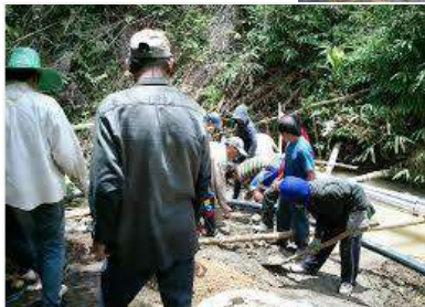
Community involved in project construction
