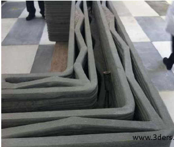
3D printed wall
