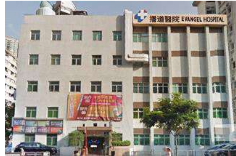
Before installation of elevator
