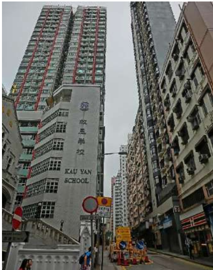
Lechler Court above Kau Yan School
