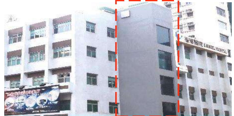
After installation of elevator
